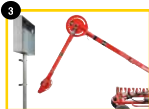
3 Align with conduit, properly adjust booms
